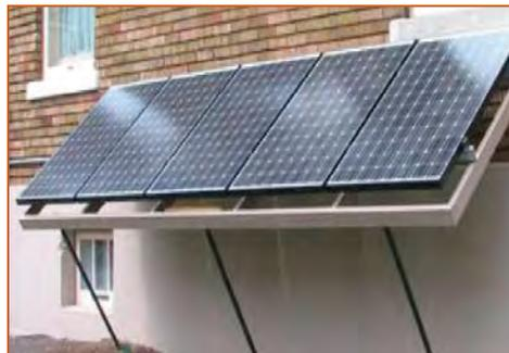
1 kW wall-mounted solar array
