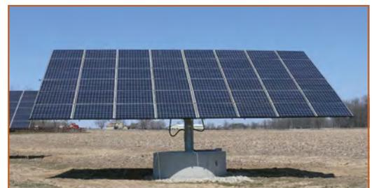
2 kW ground-mounted solar array
